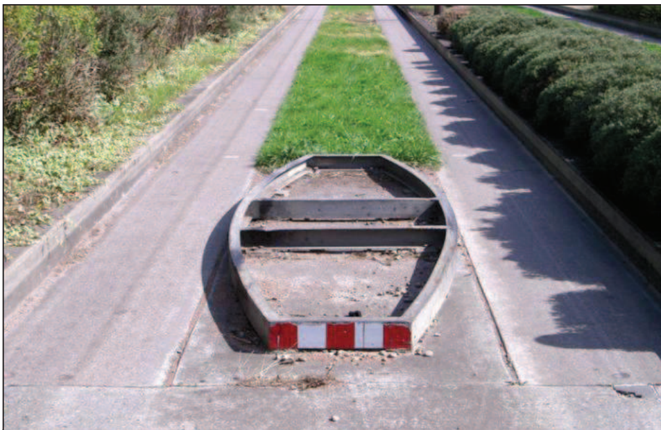
Figure 9.4 – Example of a sump buster (the width of the raised island prevents cars from passing)
