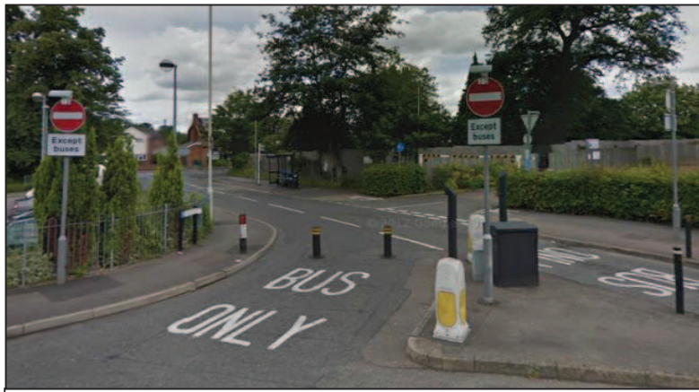
Figure 9.3 – Bus gate with rising bollards in Knaphill, Woking
